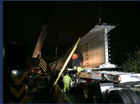
Elevated Work Approaching OVS
