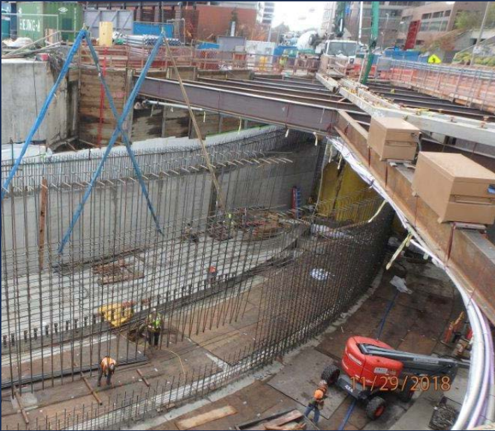
Concrete work at the North Portal (110 th )
