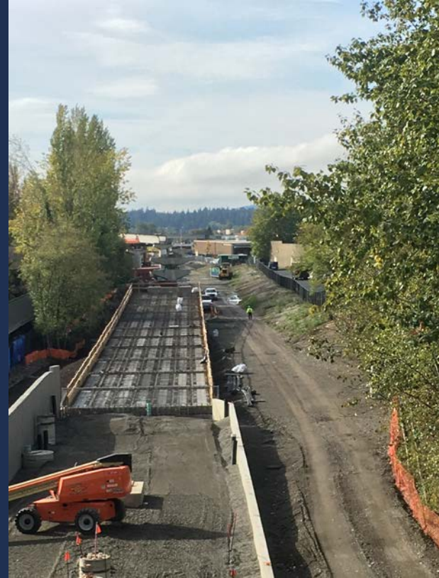
Guideway construction - trestle
