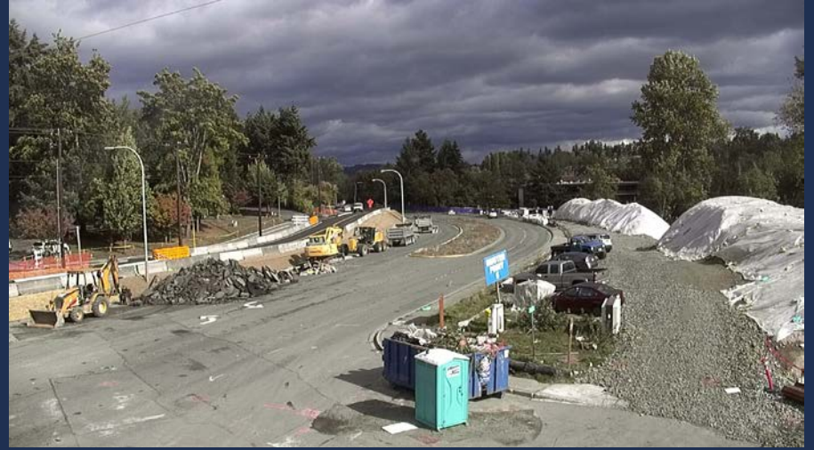
Construction of Rail undercrossing on 112 th Ave SE
