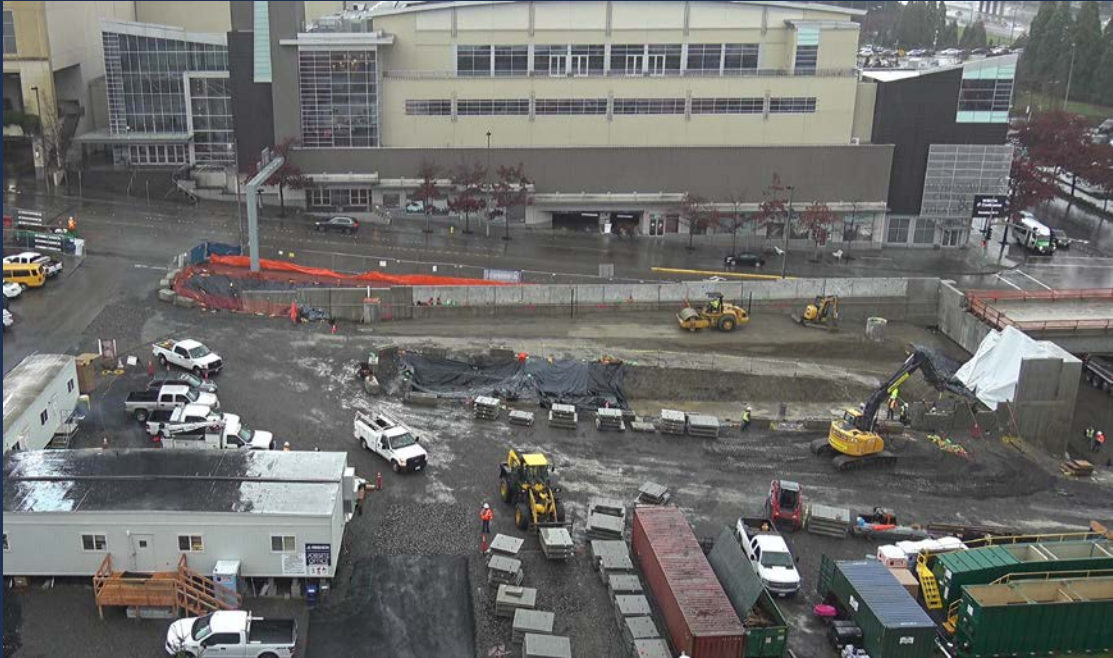
Sitework at the Station
