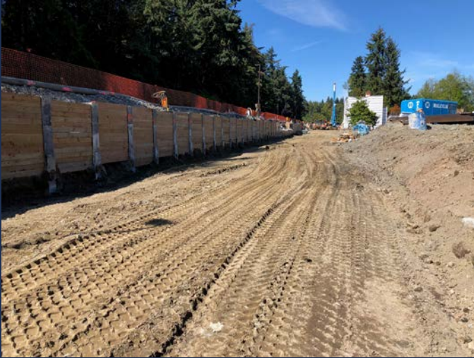
Guideway trench along Bellevue Way SE
