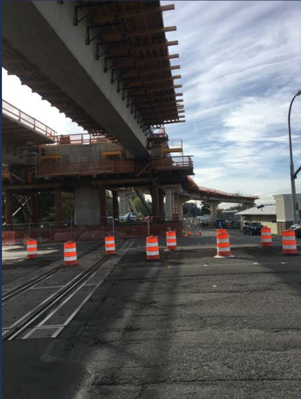
Elevated guideway over NE 8 th St.
