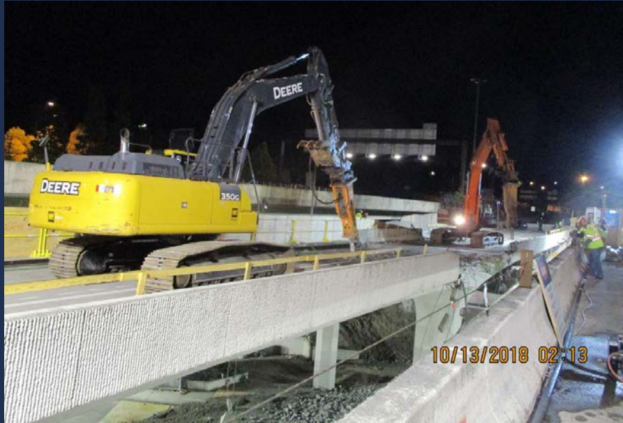
Closure and Demolition of the D2 Ramp Flyover Stop
