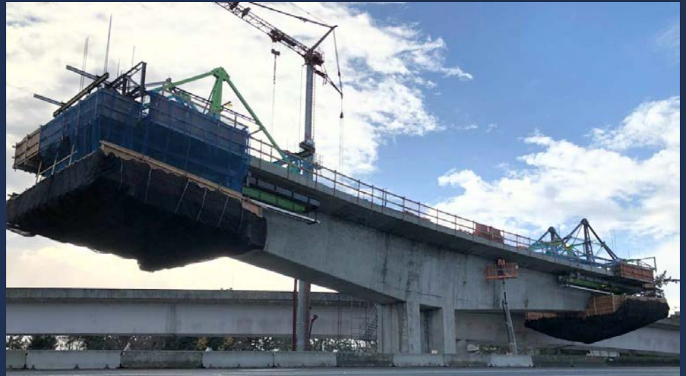
Balanced Cantilever Construction
