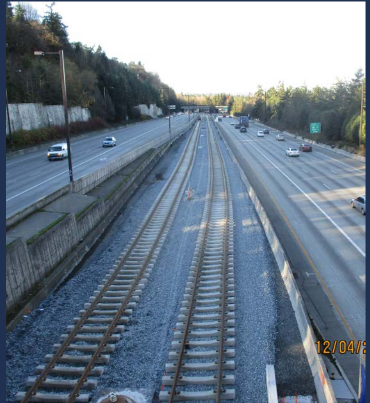
Ballasted Track on Mercer Island
