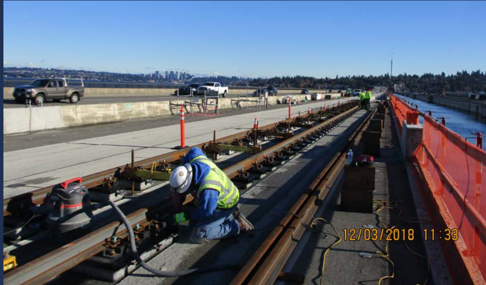
Direct Fixation Track on the Homer M. Hadley Bridge
