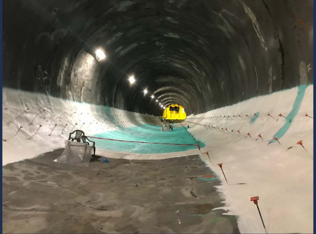
Tunnel smoothing, waterproofing and invert slab preparation
