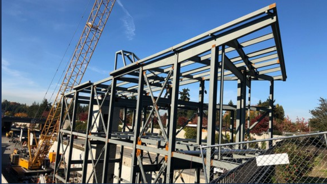
Station Entrance and Noise Walls
