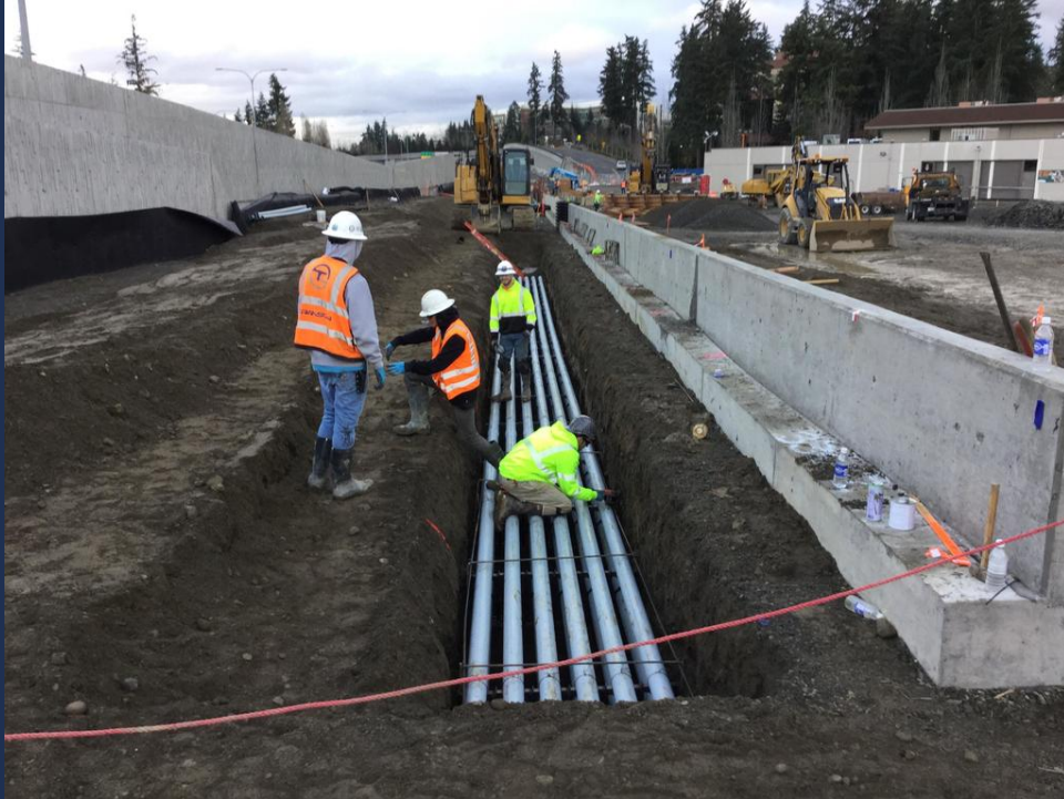
Systems Ductbank Installation
