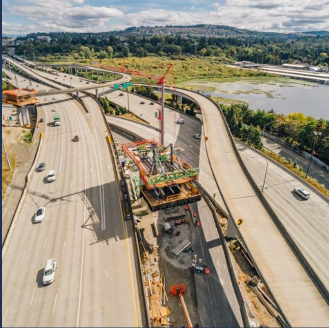
Long span construction over I-90
